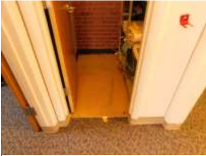
White floor tile, 6 SF, in south closet in hallway.
